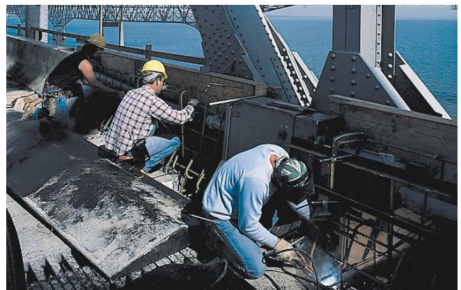
Figure 24-5 Safety clothing and/or equipment are required for some jobs.
